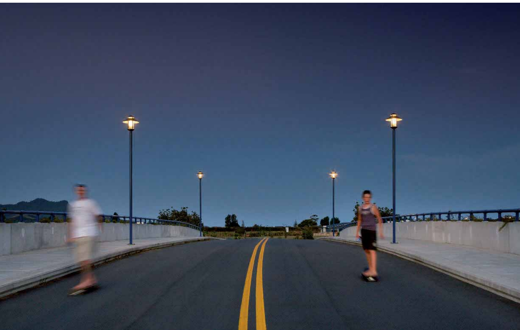
Endeavour Bridge Whitianga, Sydney (AUS).
